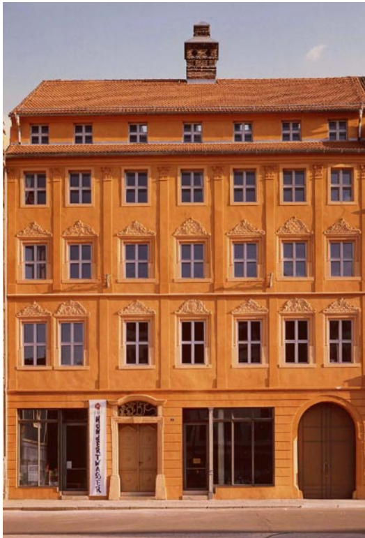
Cranachhaus Markt facade
